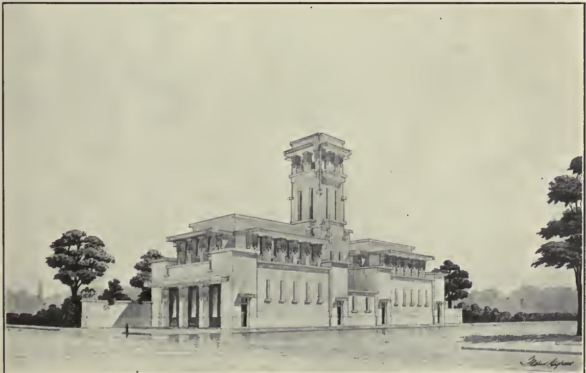
NEW FIRE AND POLICE STATION, MAISONNEUVE.
